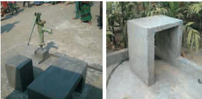
Photo 6. Accessibility adaptations for hand pump and washing area
