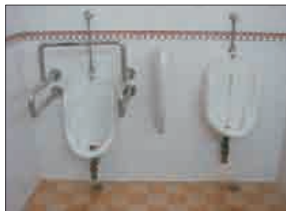
Photo 5. Urinals at two levels
