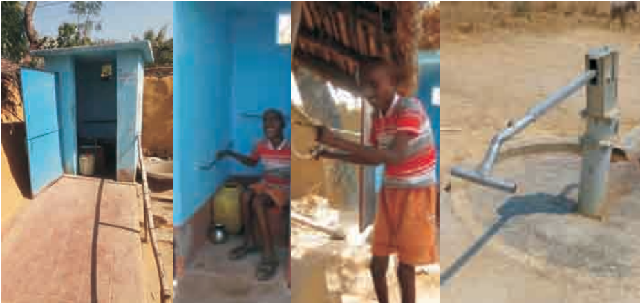
Adaptations in household toilets and handpump
