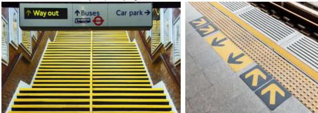
Figure 22- Brightly coloured tape on floor surface
