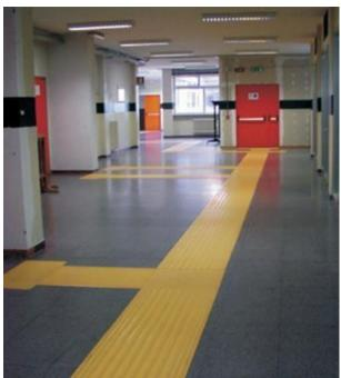
Fig.-5 Accessible Corridors and Tactile Flooring, as shown below
